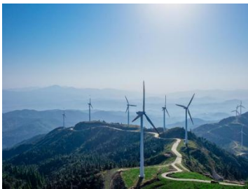
Energy and Power
